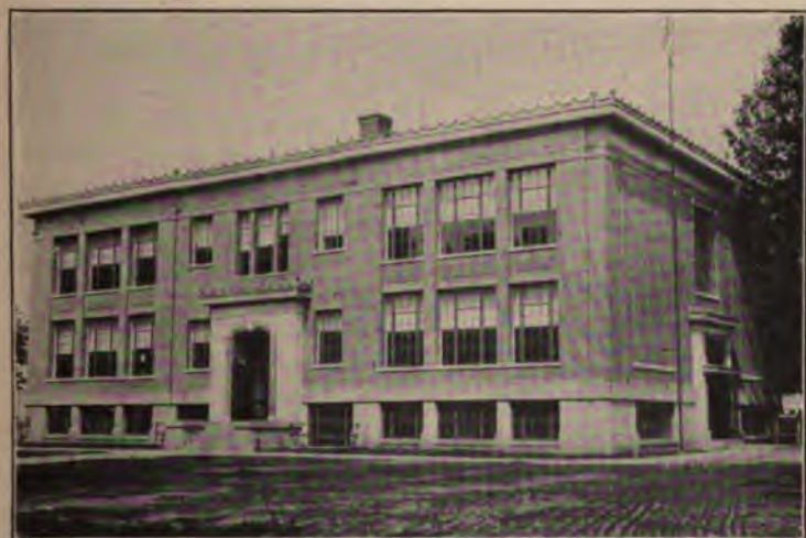
A neat example of the two-story type with basement. Poor provision for extensions
